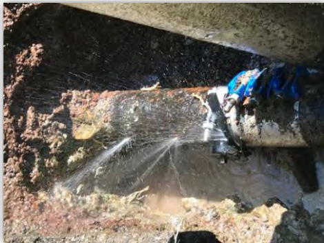
The Partnership works to upgrade waterlines to better fight fires. | TCPUD
