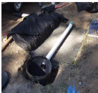
Sediment Trap and Perf Pipe over Geogrid
