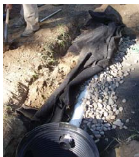
Filter Fabric and Drain Rock Cover
