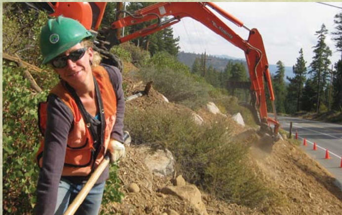
Brockway Summit Erosion Control Project, fall 2009.
